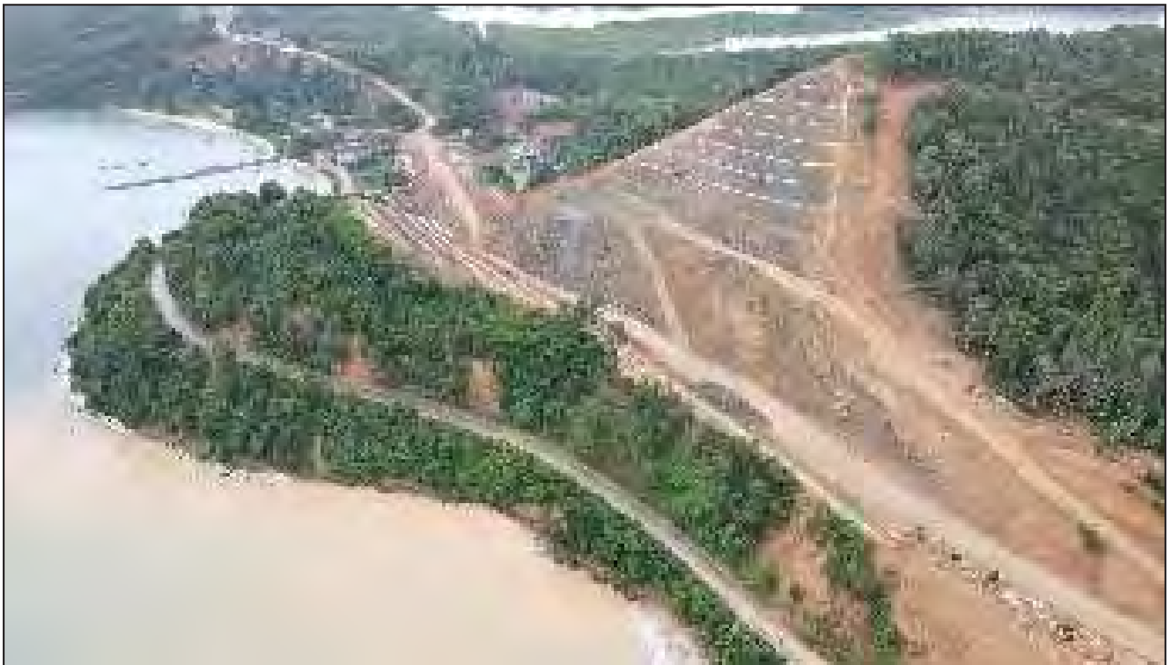
Extensive hill cutting for the new 2-lane PBH near Kampung Kastam
